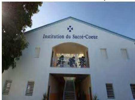
Temporary Location in Turgeau
